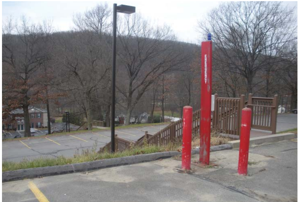
Graphic 8.25 Photograph of Steps Linking the Upper and Lower Bays of the Parking Lot to be Enhanced by Initiative C4
