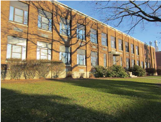
Figure 1: Davis Hall viewed from the west
