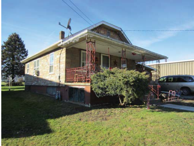
Figure 1: 206 Wilson Avenue exterior view
