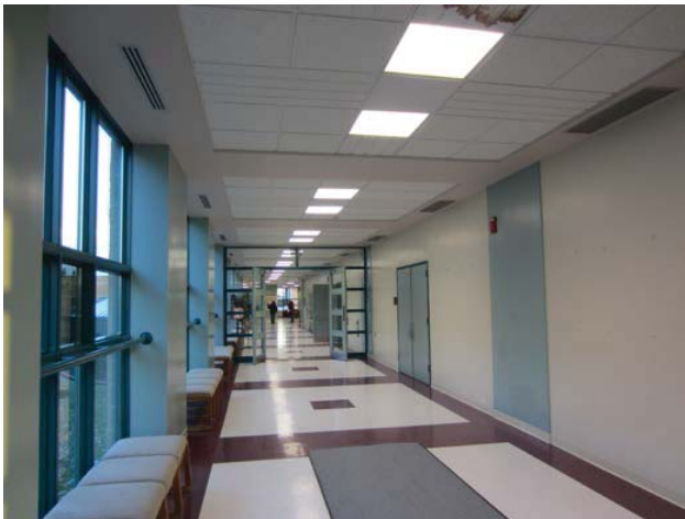
Figure 3: Typical finishes at entry corridor
