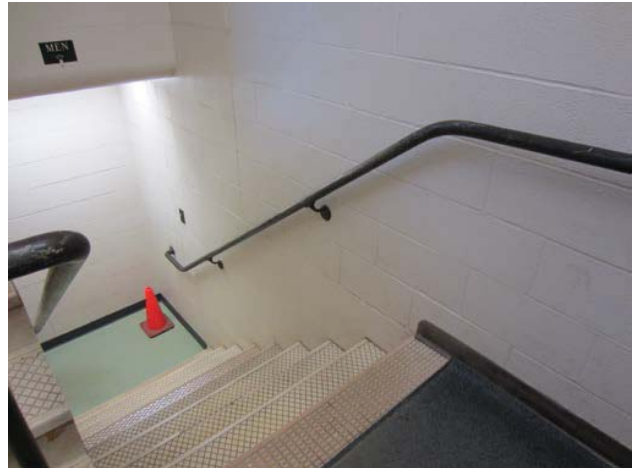
Figure 6: Stair Between Building Levels
