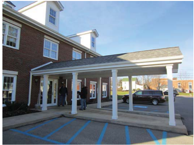
Figure 2: East façade of building with loggia
