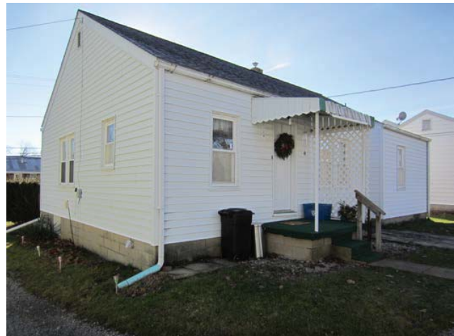
Figure 2: Building rear, exterior finishes
