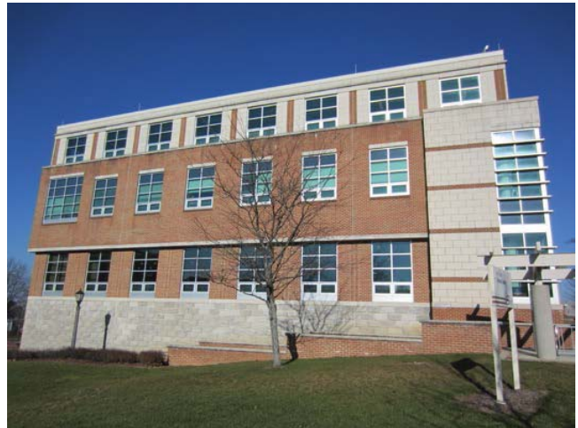
Figure 2: South façade of Carlson Library
