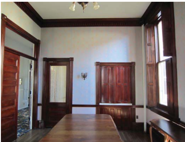
Figure 3: Typical room finishes
