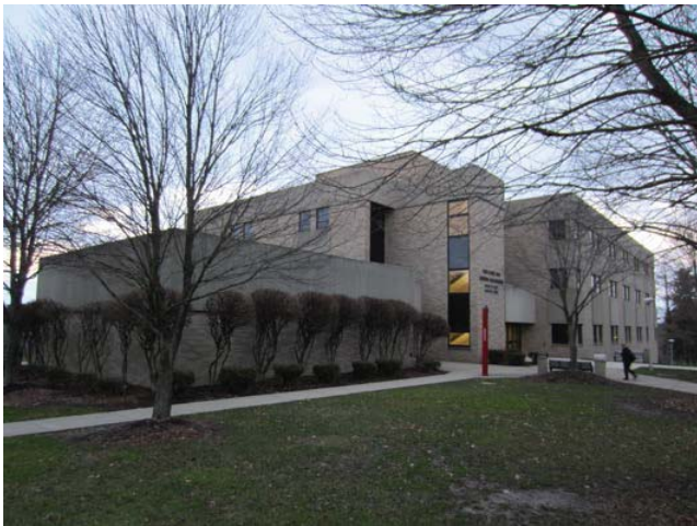
Figure 1: North and west facades of Still Hall
