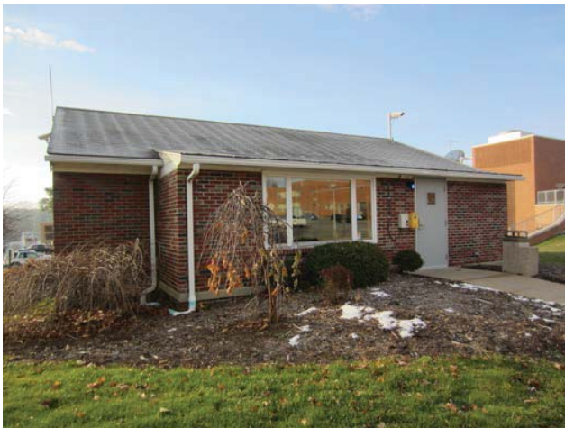
Figure 1: North facade of building
