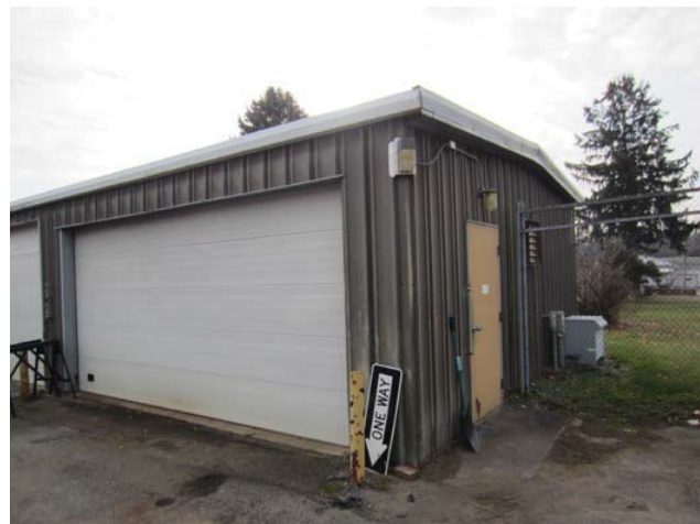
Figure 4: Northwest corner of building
