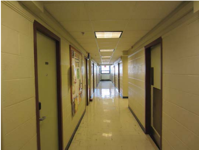
Figure 5: Interior corridor, typical finishes
