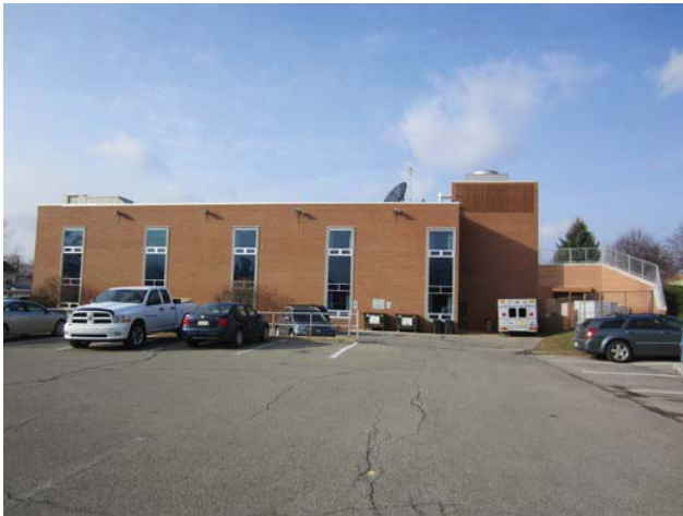
Figure 1: Becker Hall viewed from the east
