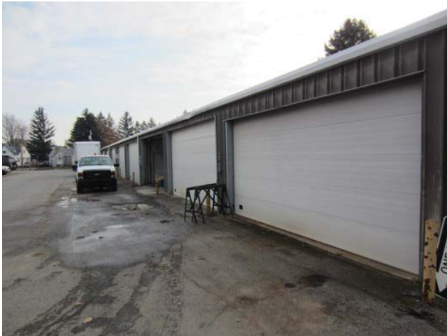
Figure 1: North façade of McEntire Warehouse
