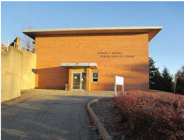
Figure 1: South facade of Keeling with retaining wall in hillside
