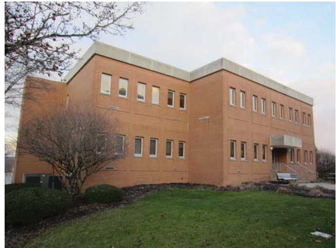
Figure 2: South façade of building, with first floor entrance
