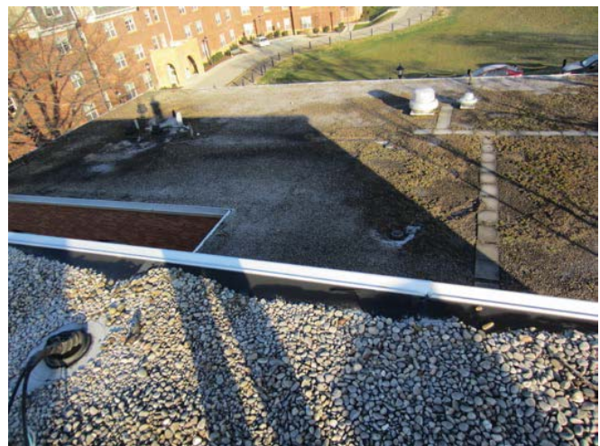
Figure 8: Plant growth on lower roof, beyond
