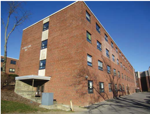
Figure 1: Givan Hall east façade with basement floor at grade
