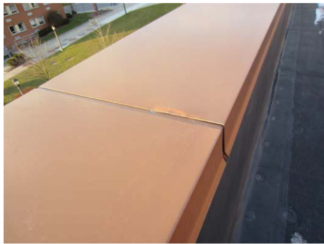
Figure 4: Membrane roofing and aluminum coping
