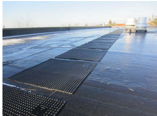
Figure 4: View of membrane roofing
