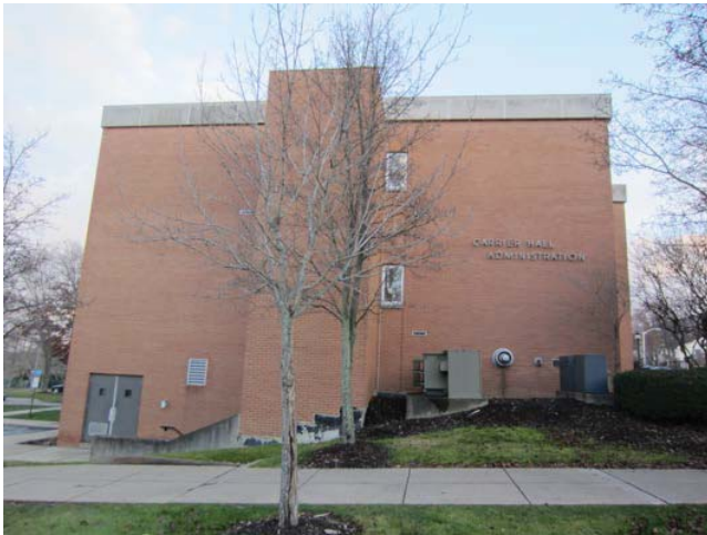
Figure 1: West façade of Carrier Administration Building, illustrating site slope
