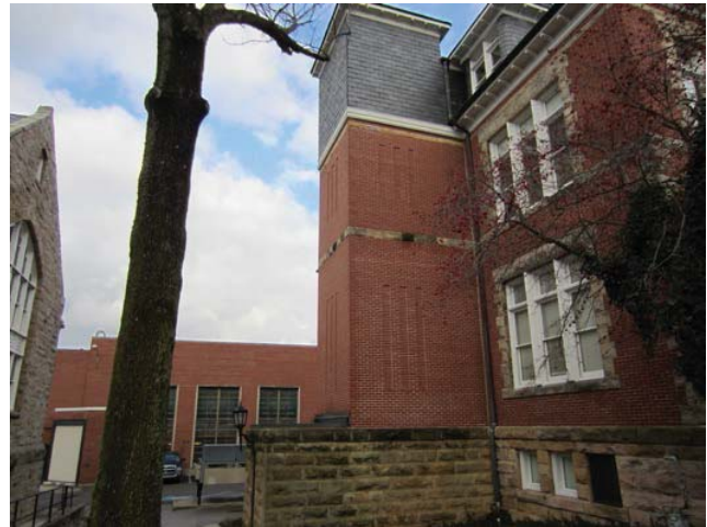
Figure 2: Elevator tower addition to west facade
