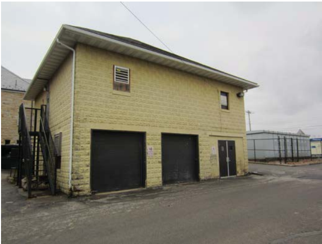
Figure 1: North façade of Sculpture Studio
