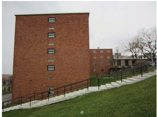
Figure 2: East façade of building
