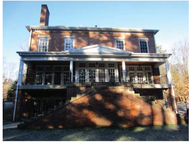
Figure 2: East façade of the building
