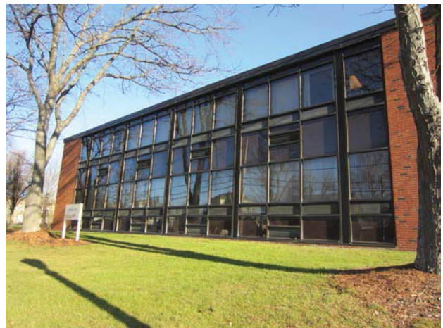
Figure 2: West façade curtain wall enclosure
