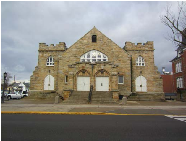
Figure 1: South façade of Hart Chapel
