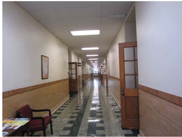
Figure 2: View of interior corridor with typical finishes
