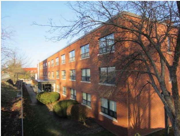
Figure 1: South façade of Ballentine Hall, from top of retaining wall
