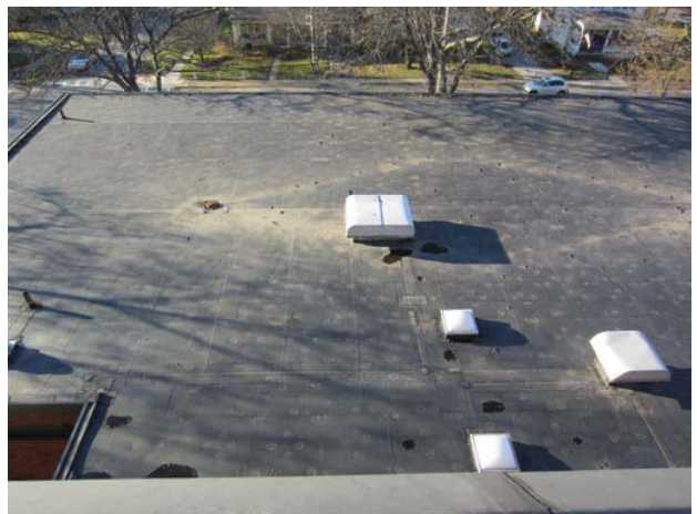
Figure 4: Membrane Roof at Annex
