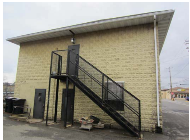
Figure 4: East façade of building
