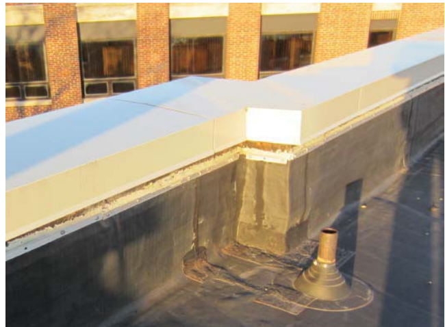
Figure 6: Roof construction with flashing bar below coping
