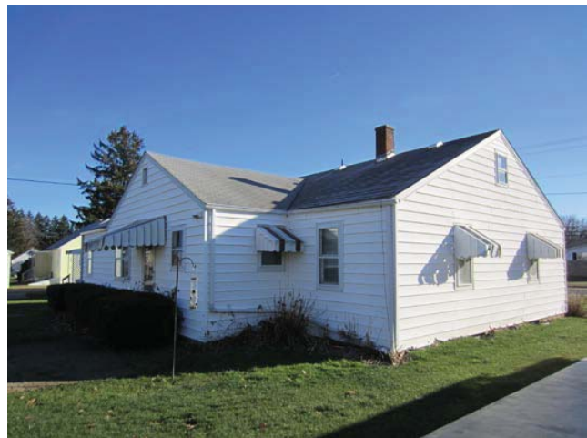
Figure 2: Building rear, exterior finishes
