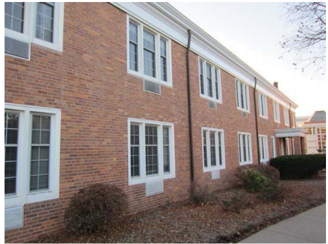
Figure 2: North façade of building
