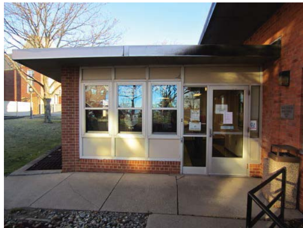
Figure 2: Reception entrance on west side of the building
