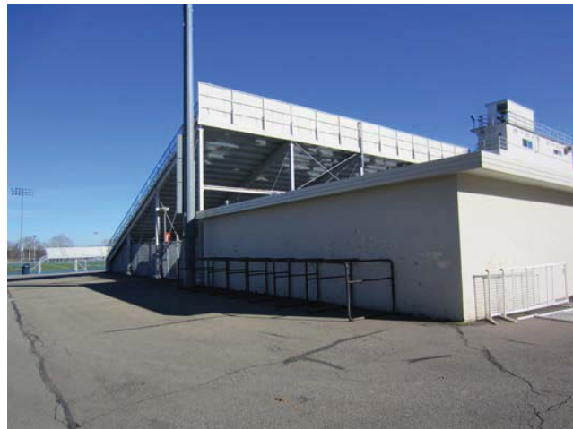
Figure 2: Locker room in foreground, with stadium beyond
