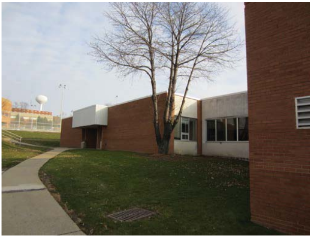
Figure 1: McEntire Entrance and Exterior Enclosure
