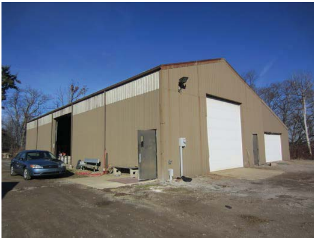
Figure 1: Pole barn exterior view
