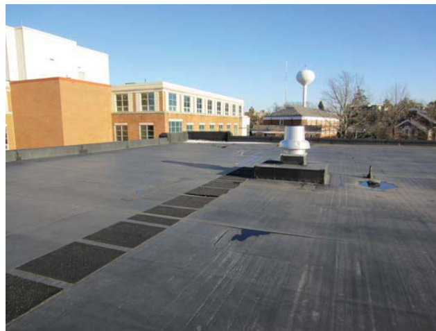
Figure 4: View of membrane roofing
