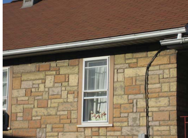
Figure 2: Building exterior finishes
