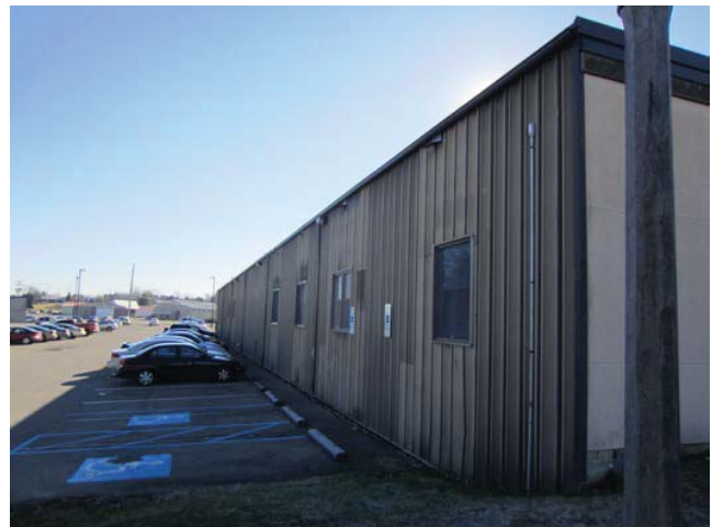
Figure 2: North façade of building
