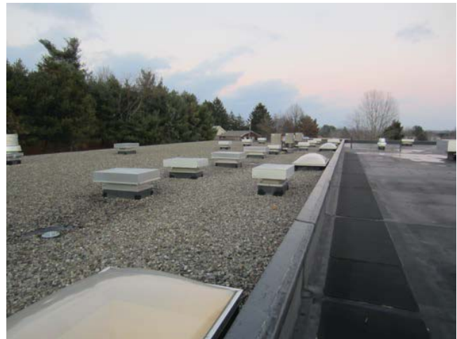
Figure 6: Membrane roof assemblies, with and without ballast
