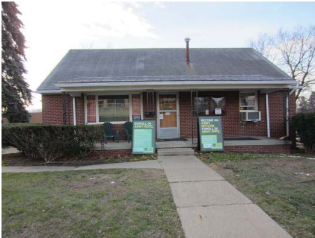
Figure 1: North facade of building
