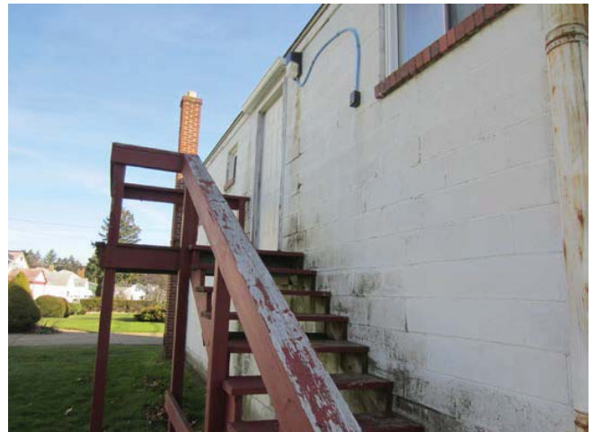
Figure 2: Building exterior finishes
