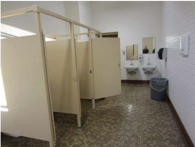
Figure 5: View of typical toilet room
