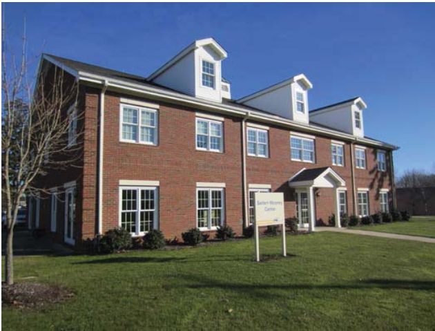
Figure 1: West façade of the Center for Advancement
