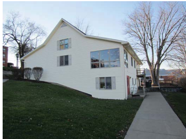
Figure 2: East and north facades of building
