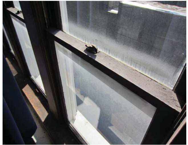
Figure 6: Typical operable wood and glass window
