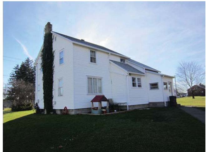
Figure 2: Building rear, exterior finishes
