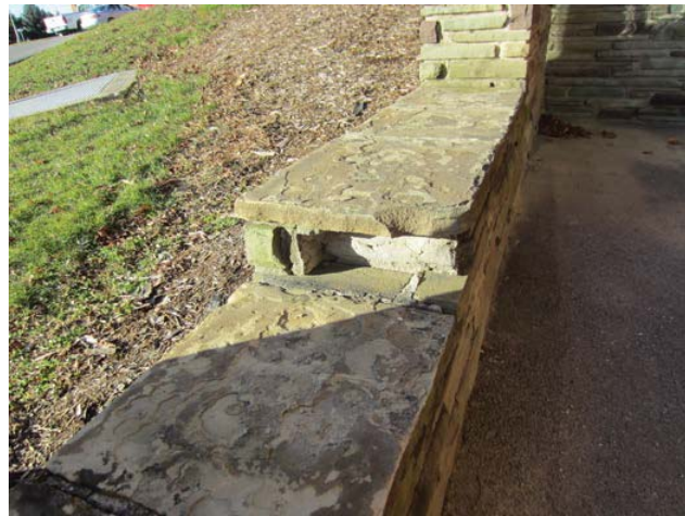
Figure 2: Fieldstone wall conditions at entrances (typical)
