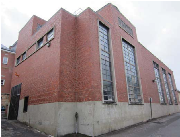
Figure 1: Northeast corner of Utility Plant
