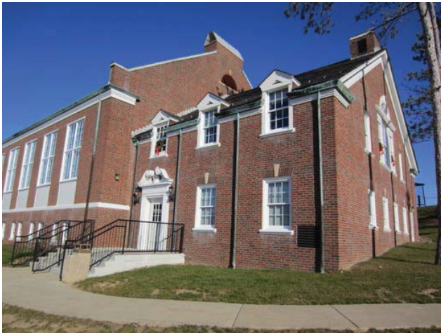
Figure 1: South and east façades of Harvey Hall
