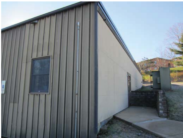
Figure 1: Northwest corner of building, with entrance beyond
