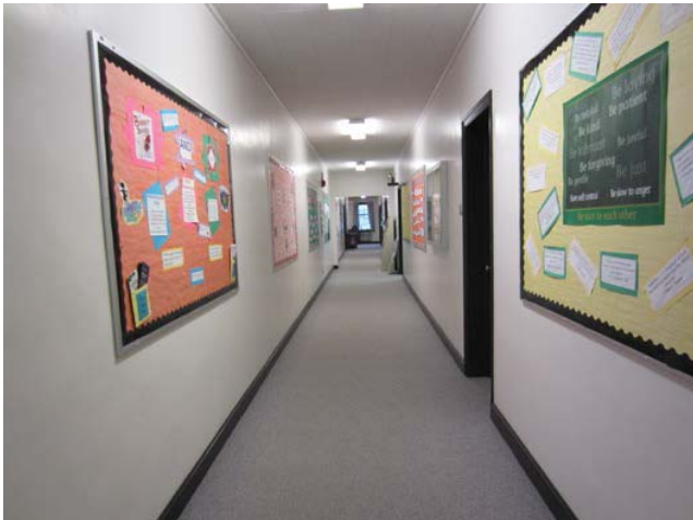
Figure 3: Interior corridor finishes
