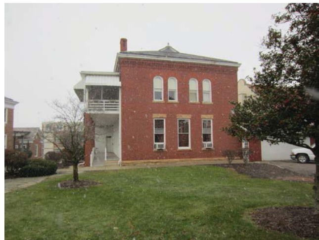
Figure 4: East elevation of building, with porch
