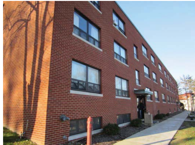
Figure 2: North façade of the building, with basement windows
