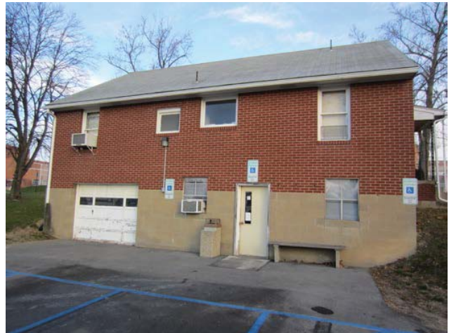
Figure 2: South facade of building
