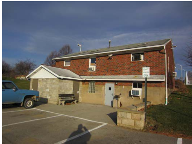
Figure 2: South facade of building
