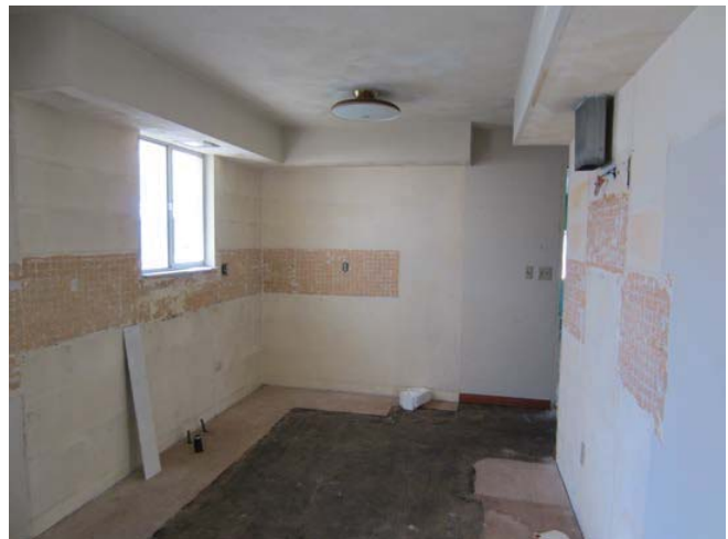
Figure 2: Interior view of former kitchen
