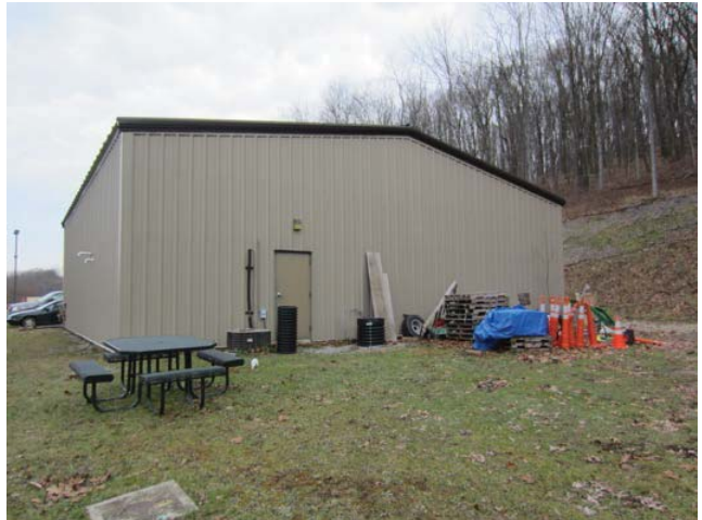
Figure 2: Pole barn exterior view from south
