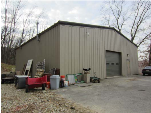
Figure 1: Pole barn exterior view from north
