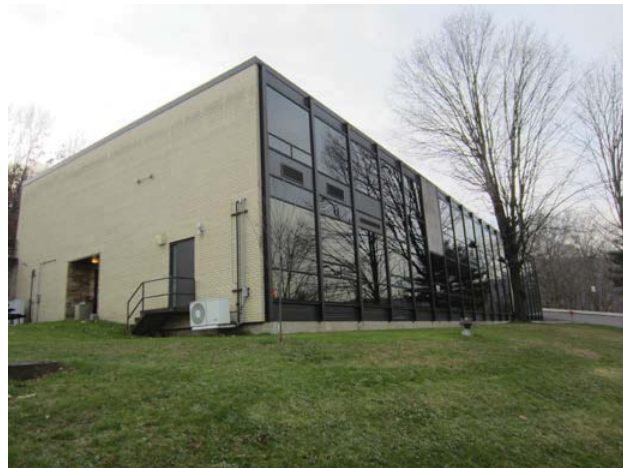
Figure 2: West façade curtain wall
