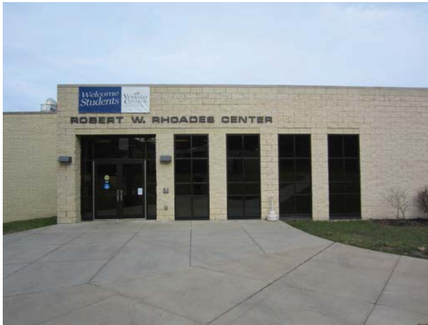
Figure 1: Rhoades Center Entrance
