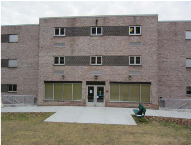
Figure 1: Montgomery Hall east elevation
