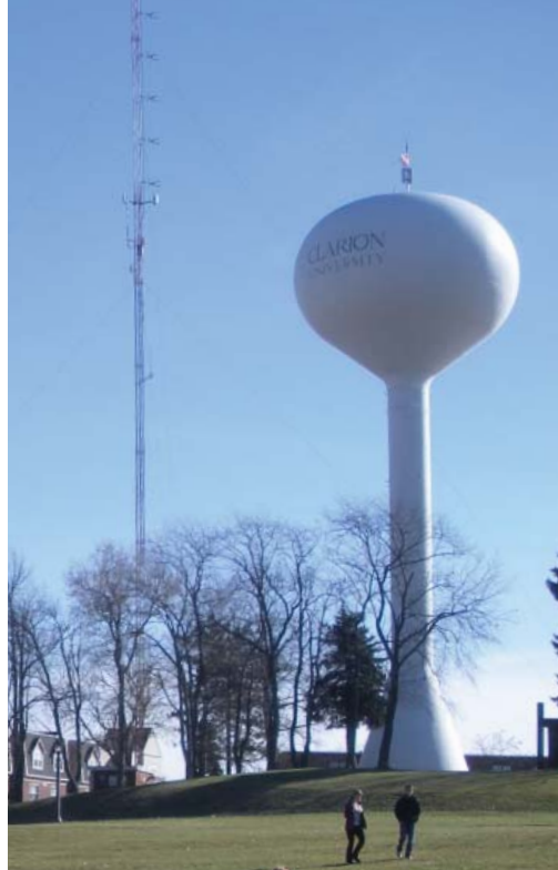
Graphic 3.21 Communications And Water Tower
